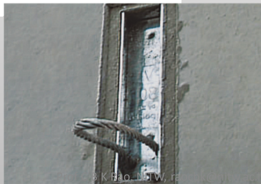
TYPICAL CROSS WALL DETAIL(SHEAR LOOP)
